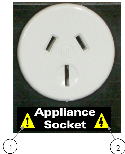
Figure 1.2-1 High Test Voltage at Appliance Socket
